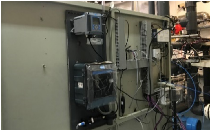
Figure 1. Installation point for Hach ULR CL17sc on a side of the GAC tank (left) and sc1000 controller displaying chlorine concentrations from both CL17 and ULR CL17sc analyzers (right)
